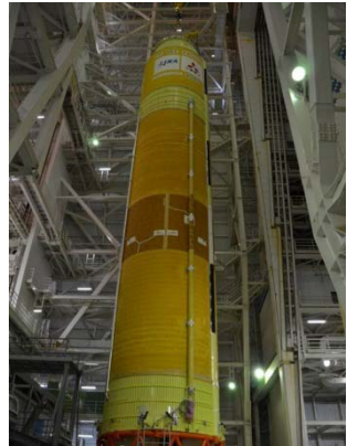
1 st stage erection
