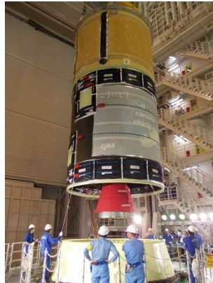
2 nd stage erection
