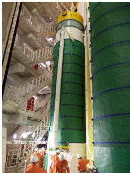
SRB-A installed (completed on Mar. 24, 2012)
