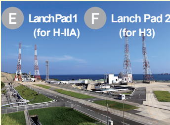
Launch Vehicles are transported from the VAB to the Launch Pad right before the launch. H-IIA Launch Vehicles are launched from the Launch Pad 1 and H3 Launch Vehicles are launched from the Launch Pad 2.
